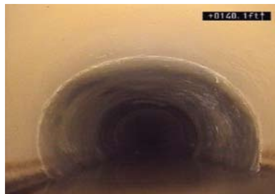
SEWER LINE AFTER CIPP POINT REPAIR
