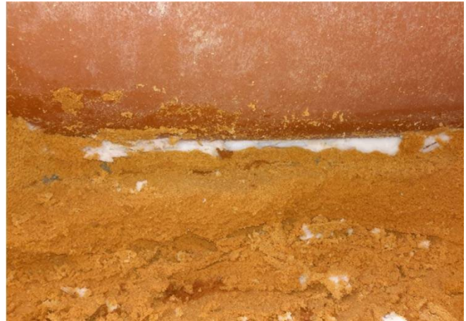
Figure 92: Neat Grout Continues Along Pipe in Voided Area
