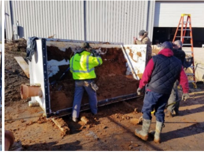
Figure 133: Removal of Trench and Backfill
