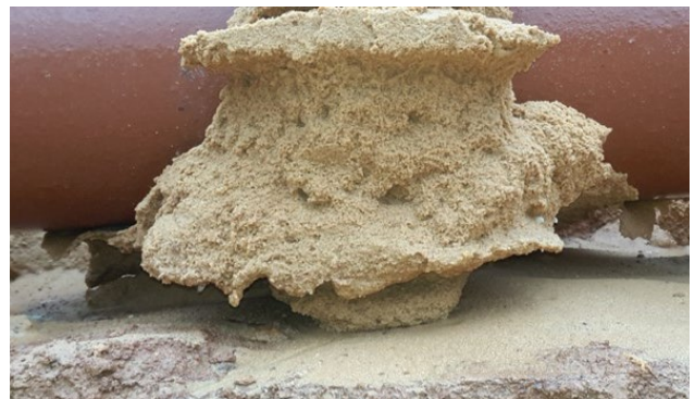
Figure: 104: Defect B: 23 Second Gel Time
