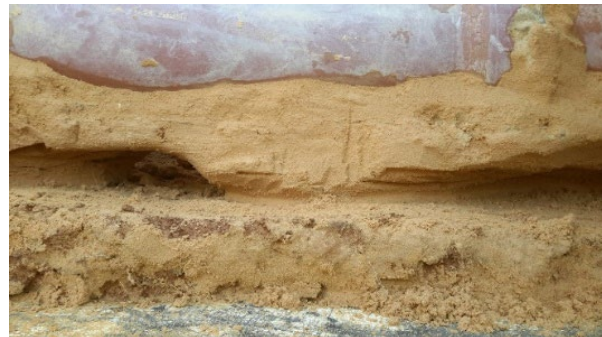
Figure 79: Location of Grout Below Structure
