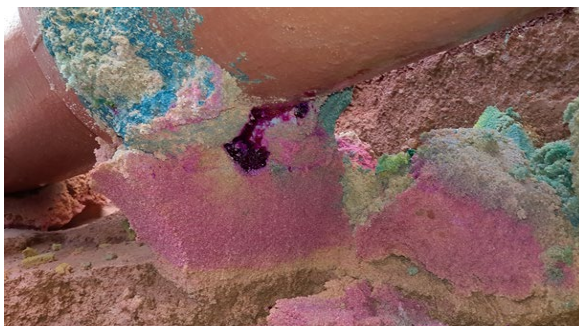
Figure 49: Neat Red Grout Observed Below Pipe
