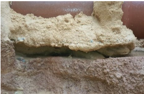
Figure 96: Longitudinal Support of Pipe
