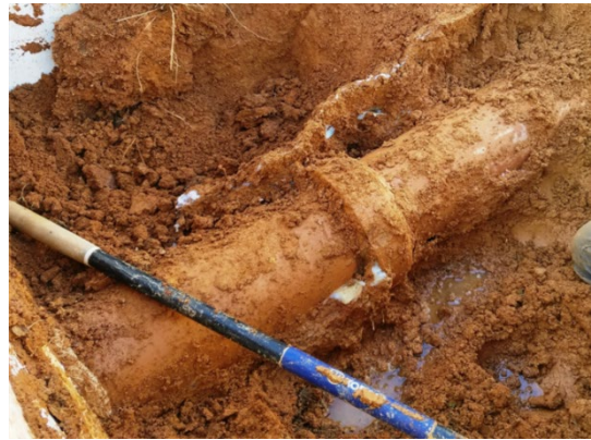
Figure 139: Grout Installed in Clay Backfill
