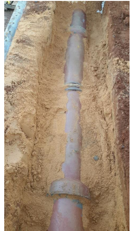
Figure 62: Pipe with Defects Installed In Sand Bedding
