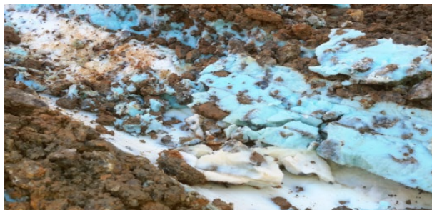
Figure 123: Section of Neat Grout Below Pipe
