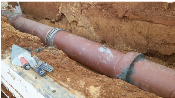
Figure 63: Pipe Installation Prior to Backfill
