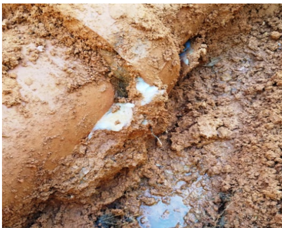
Figure 188: Neat Grout Seal at Defect
