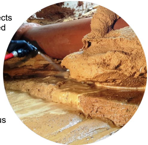
Figure 18: Water Used to Remove Loose Material
