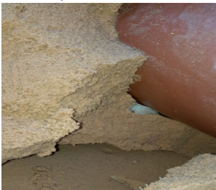
Figure 73: Neat Grout Below Pipe
