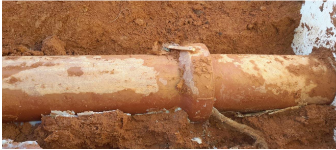
Figure 140: Neat Grout Along Bottom of Pipe
