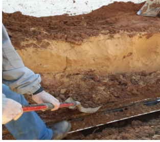
Figure 17: Removal of Backfill
