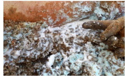
Figure 179: Stone Grout Trial
