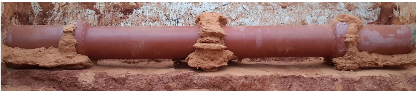
Figure 114: 23 Second Gel Time Grout Formations
