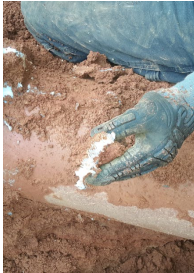
Figure 147: Neat Grout
