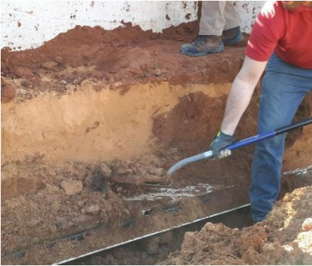
Figure 64: Removal of Loose Backfill After Grouting
