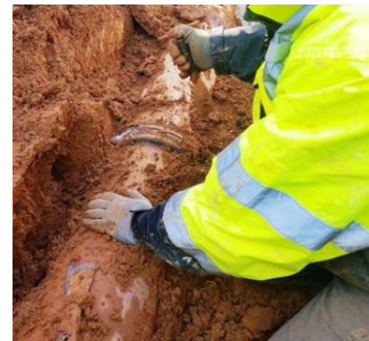
Figure 135: Removal of Clay Backfill
