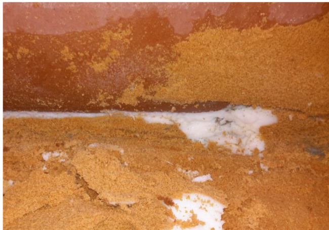
Figure 91: Neat Grout Fills Voids Below Pipe
