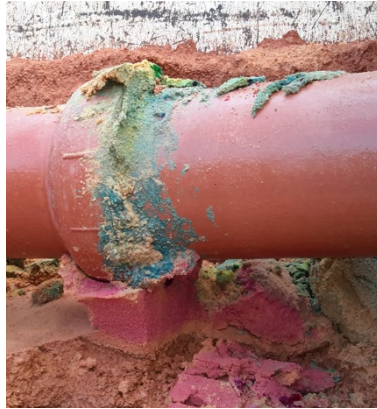
Figure 161: Colored Grout Layers
