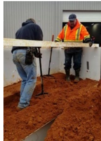
Figure 131: Tamping During Install
