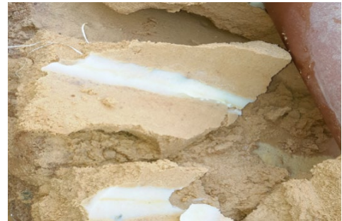
Figure 85: Neat Grout Within Bridge
