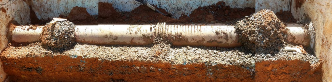
Figure 172: 24 Second Gel Time Grout / Stone Matrix
