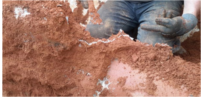
Figure 142: Neat Grout Fin
