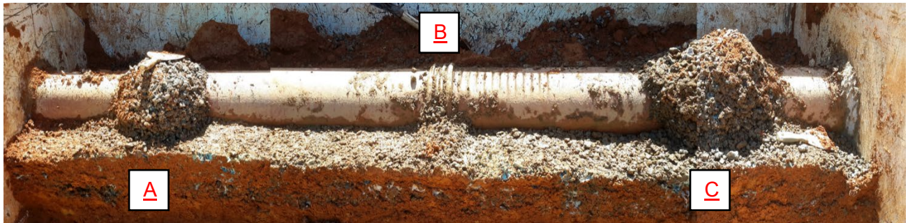
Figure 117: Grout Formation After Sealing in Stone
