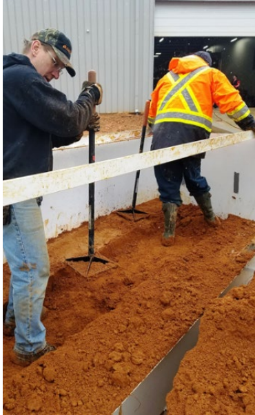
Figure 12: Hand Tamping
