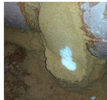
Figure 165: Neat Grout Seal
