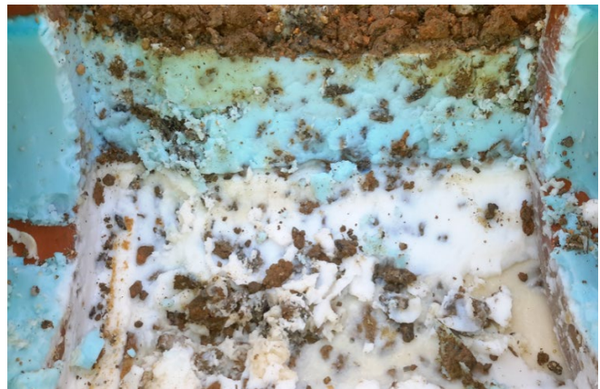
Figure 122: Pipe Removed to Reveal Grout Segment Below
