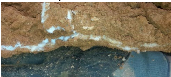
Figure 155: Segment of Grout Fin
