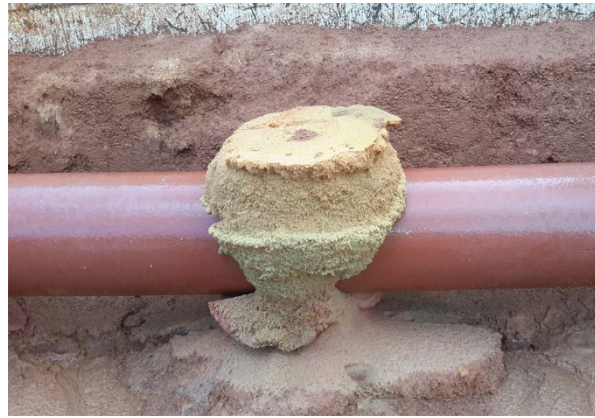
Figure 59: Side View of Grouted Mass
