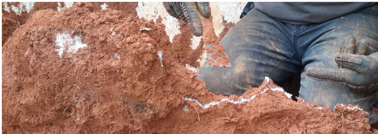
Figure 149: Grout Followed Path of Least Resistance
