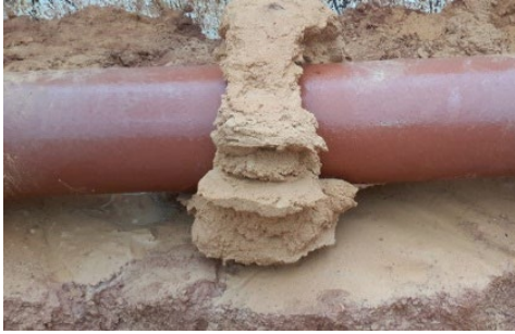
Figure 93: Fin formation front view
