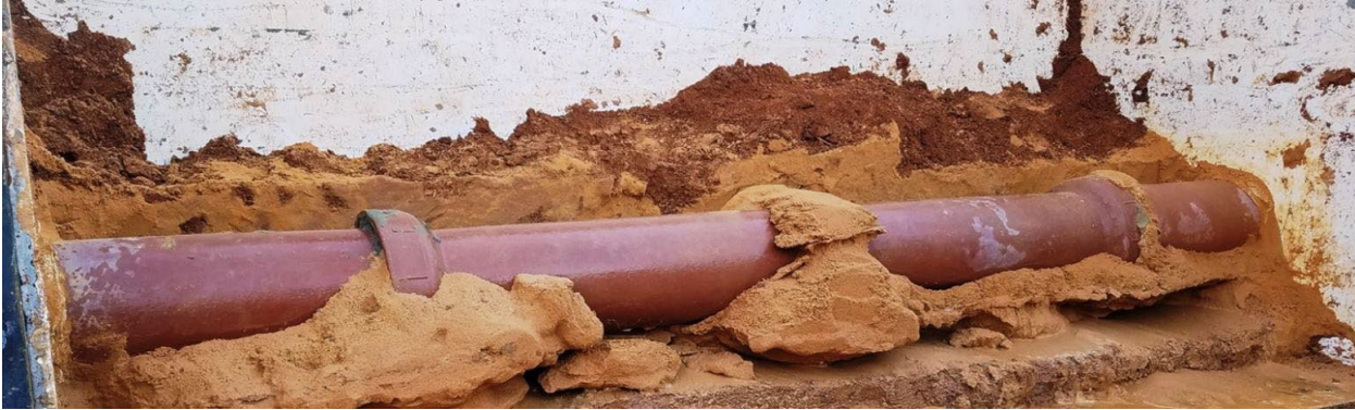
Figure 88: 55 Second Gel Time Grouted Soil Formations
