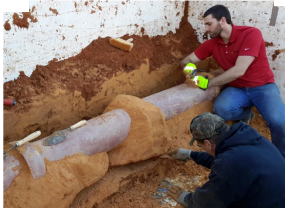
Figure 67: Full Extent of Grouted Mass Revealed
