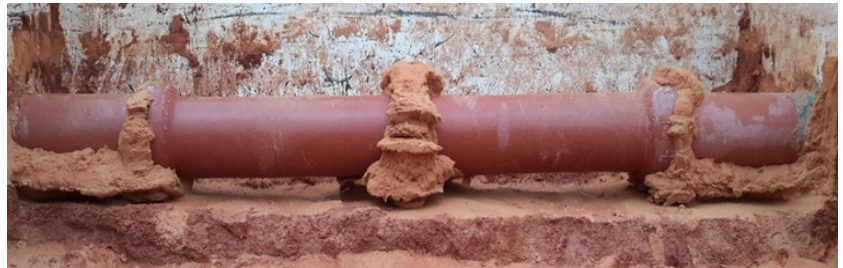
Figure 102: Test Cell Grout Formation Using 23 Second Gel Time
