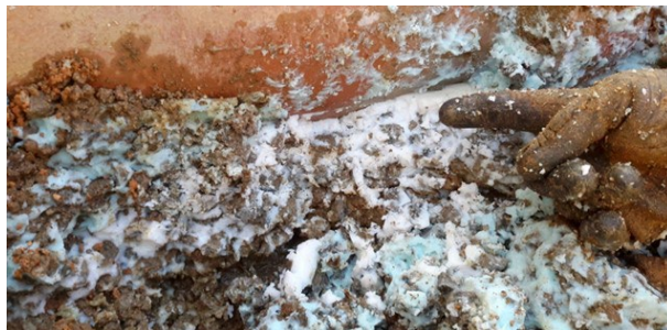
Figure 121: Neat Grout Filling Void Below Pipe
