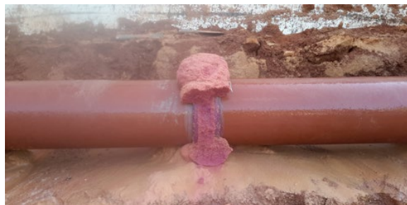
Figure 56: Side View Grout Mass
