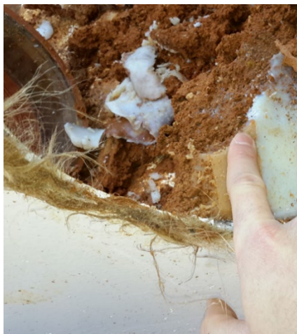
Figure 136: Neat Grout Segments
