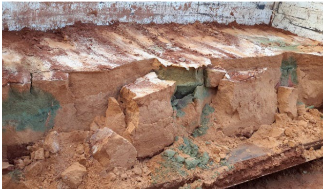
Figure 20: Colored Grouted Formation First Revealed
