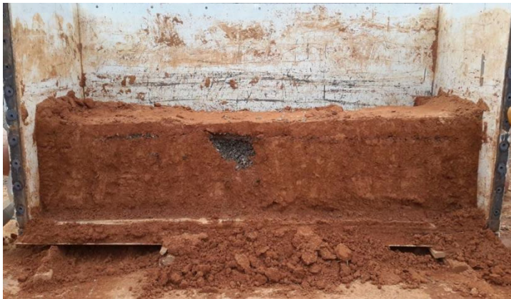
Figure 116: Test Cell After Grouting In 57 Stone
