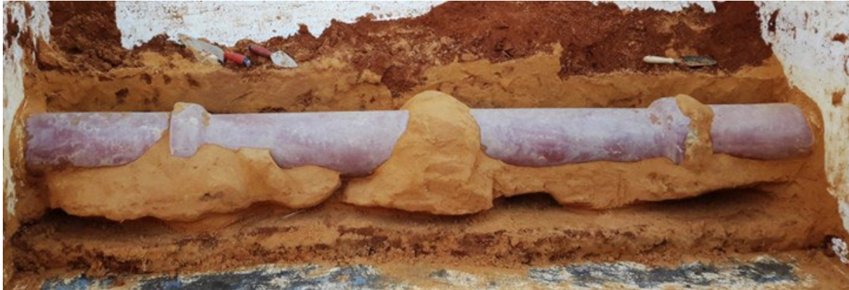
Figure: 115: 55 Second Gel Time Grout Formations
