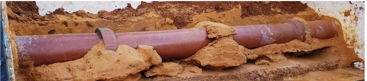
Figure 113: 55 Second Gel Time Grout Formations
