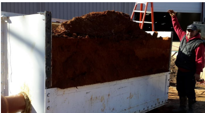
Figure 16: Superior Plate of Test Cell Removed After Grouting
