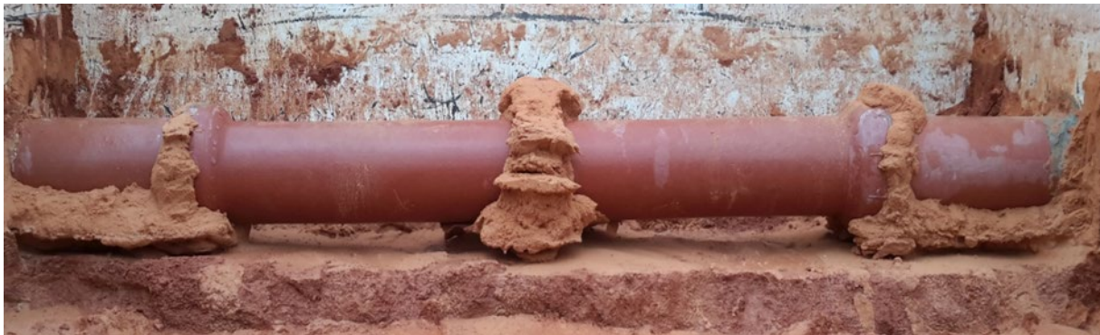
Figure: 106: 23 Second Gel Time Grout Formations
