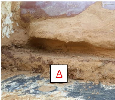
Figure 80: Grouted Formation at Defect A
