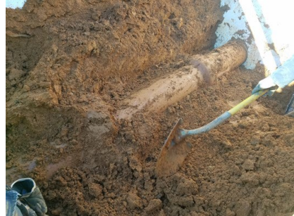
Figure 134: Reveal of Pipe After Grout
