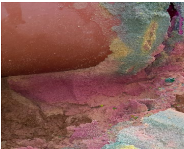
Figure 55: Grouted Mass Below Pipe
