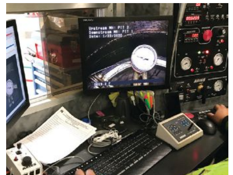
Air testing and Sealing Mainline
