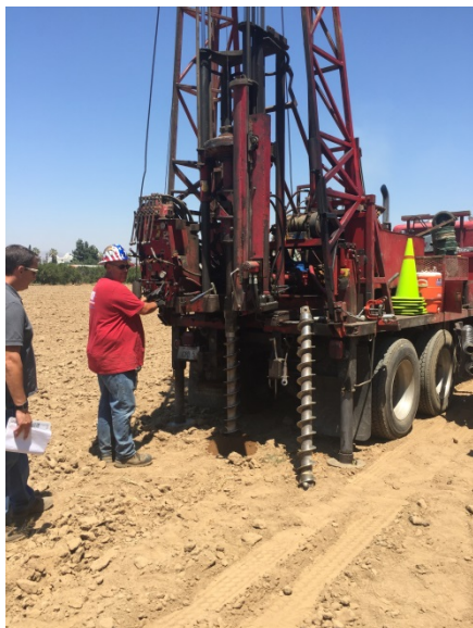
Image 1. Standard drill rig used to produce borehole to depth of 20 ft.
