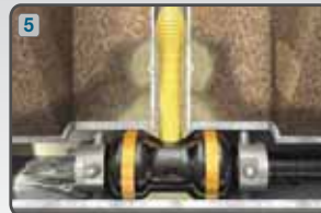
Lateral packer injecting grout
