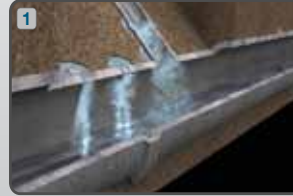
Leaking lateral
