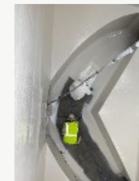
Figure 2. Applying a mortar resurfacer followed by a resinous lining will best protect assets exposed to high turbulence and elevated H 2 S levels.
