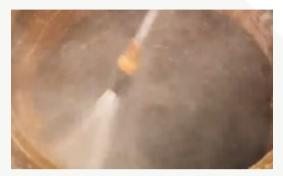
loose material, the surface is not sound. You may need to use impact tools like chipping hammers to remove unsound mortar.
